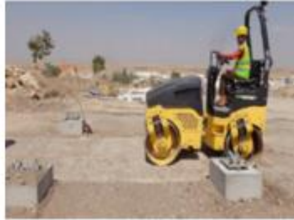
Filling For Foundation
